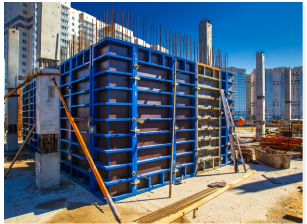
LIFT SHAFT FORMWORK
