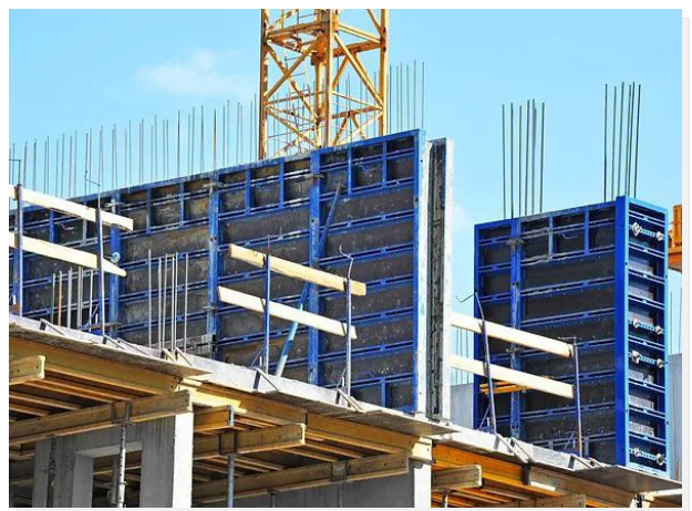
SHEARING WALL FORMWORK
