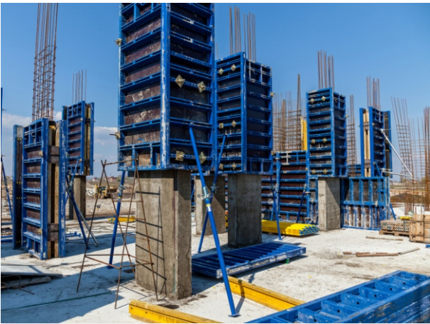
COLUMN FORMWORK
