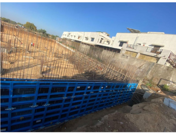
WALL FORMWORK
